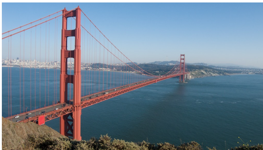
Figure 1: Golden Gate Bridge: Gateway to San Francisco Bay
